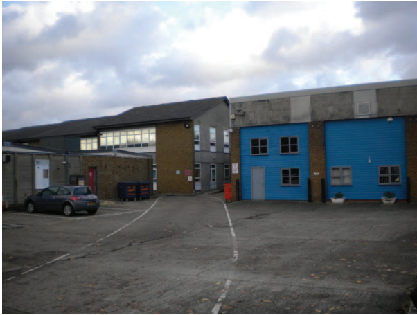
A.7 North Block offices (rear left) & vehicle workshop (righthand side)
