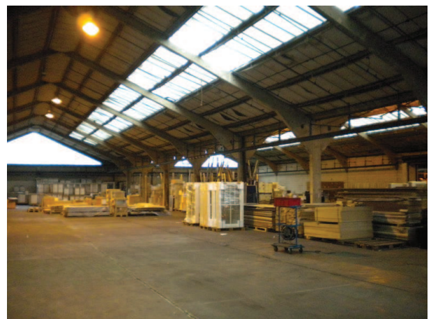
A.6 Inside the main warehouse
