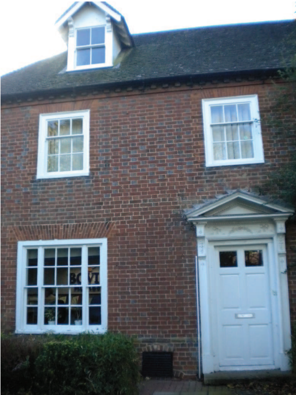
C.3 The listed element of the Manor House
