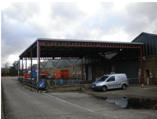
A.5 Eastern side of the main warehouse
