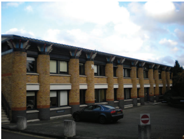
A.3 Main office building
